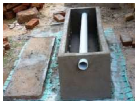
Figure 30: Aeration chamber of Iron Removal Plant
